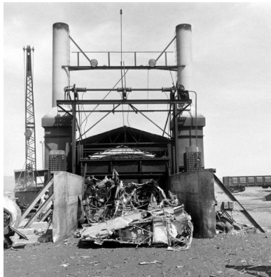
3. One of the three smelters, or furnaces, used at Kingman to melt small pieces of aircraft into ingots
